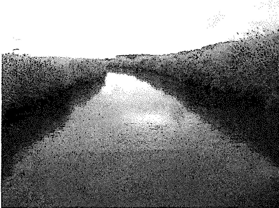
Photo 2. Eighteen feet wide channel, .5 feet deep, about 5 cfs, fine silt bottom
